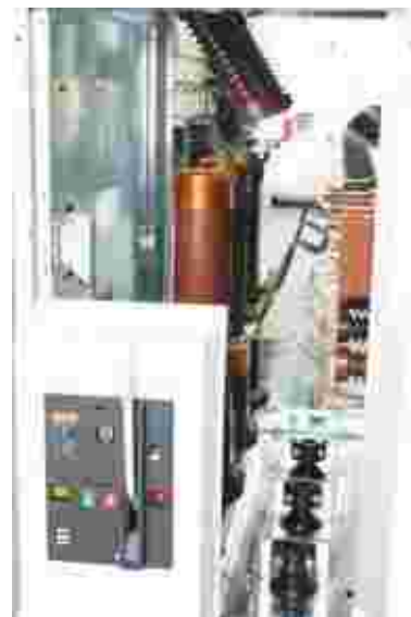
Cable Compartment of Cubicle with Circuit Breaker
